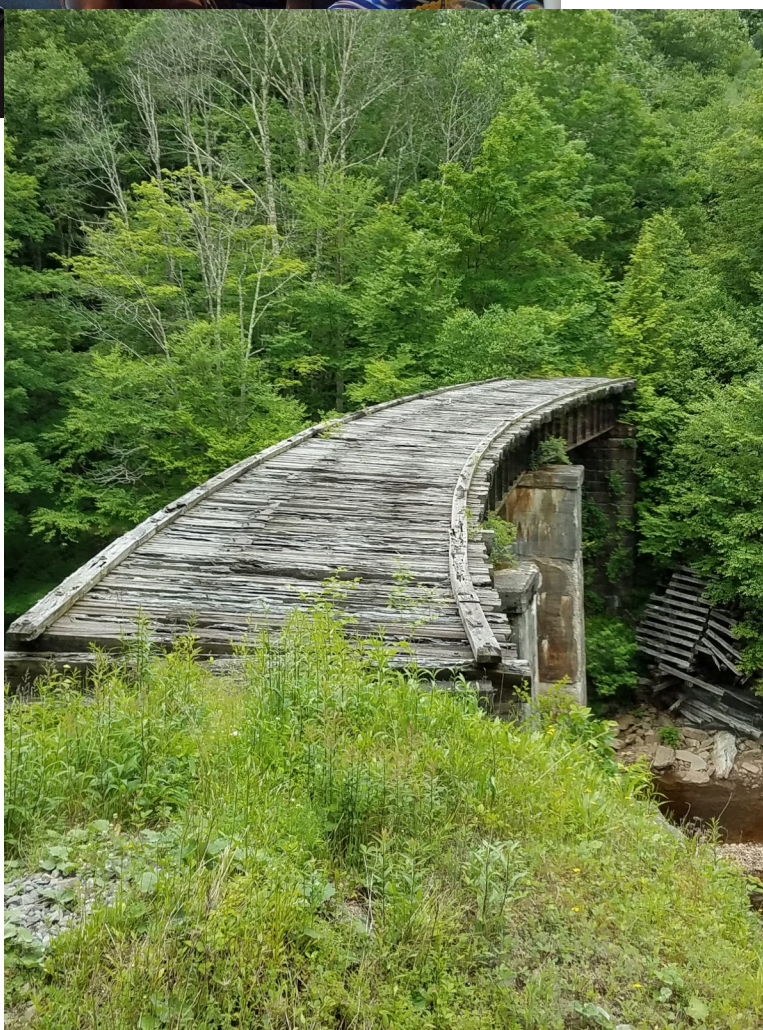
Abandoned curved deck girder bridge. Photo by John Harris
